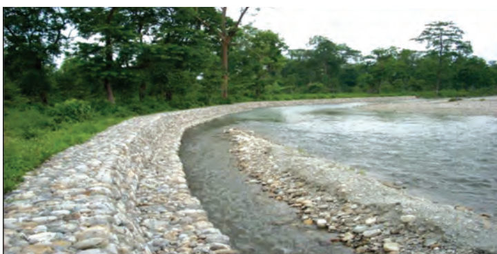
(NREGS) : Murti river bank protection work at North Indong block ( Lower Tista Catchment Range) under Jalpaiguri Soil Conservation Division
