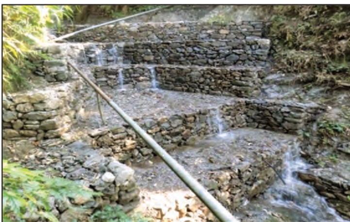
Gully Plugging works at Tankyjhora, Mahaldiram-III under RKVY Scheme over 45 m 3 2016-17 Kurseong Soil Conservation Division
