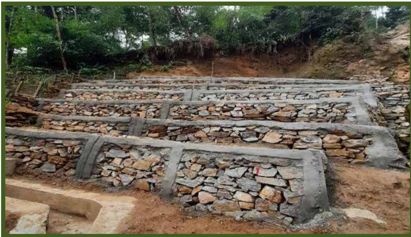
Hand packed wall of 150 m 3 at Phuguri block constructed under RKVY during 2019–20 under West Balason Catchment Range of Kurseong Soil Conservation Division
