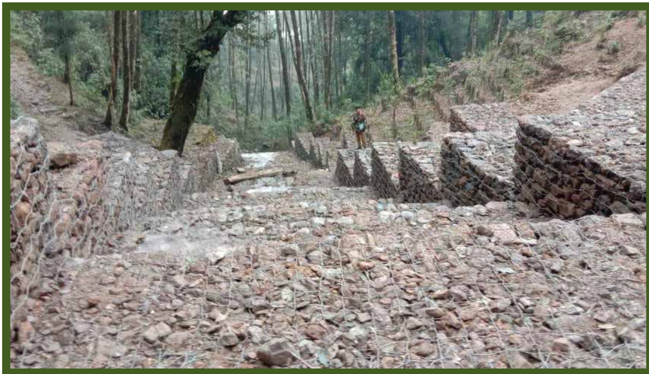
Boulder Sausage wall of 150 m 3 at Mahaldiram block-II constructed under CAMPA FUND (TLDP-IV) during 2019–20 under East Balason Catchment Range of Kurseong Soil Conservation Division
