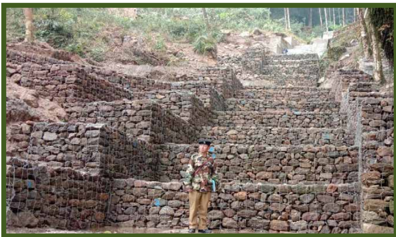
Boulder Sausage wall of 150 m 3 at Mahaldiram block-II constructed under CAMPA FUND (TLDP-IV) during 2019–20 under East Balason Catchment Range of Kurseong Soil Conservation Division
