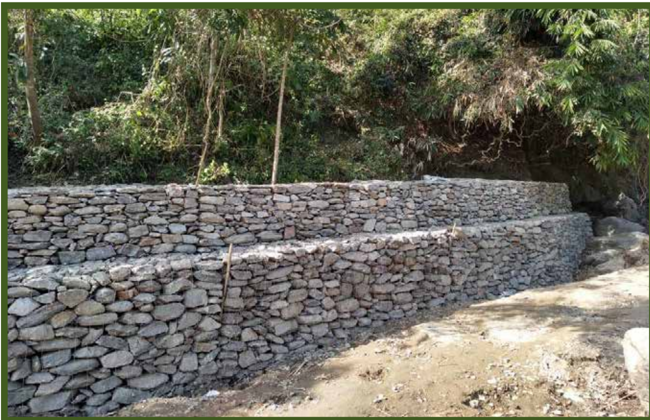
Hand packed wall of 250 m 3 at Khairbani block constructed under RKVY during 2019–20 under Lower Mahanadi Catchment Range of Kurseong Soil Conservation Division
