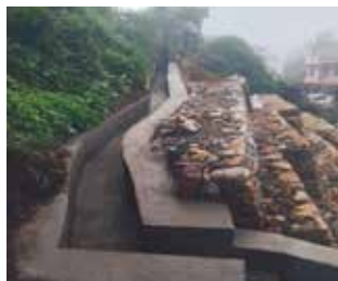
Catch Water Drain (50 rmt) at Lepcha Jagat
