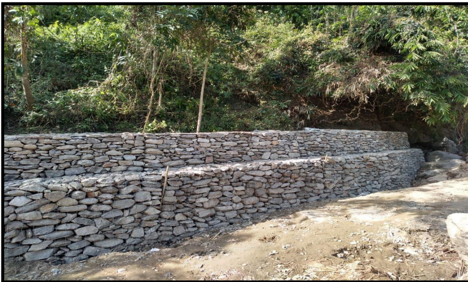
Hand packed wall of 250m 3 at Khairbani block constructed under RKVY during 2019-20 under Lower Mahanadi Catchment Range of Kurseong Soil Conservation Division
