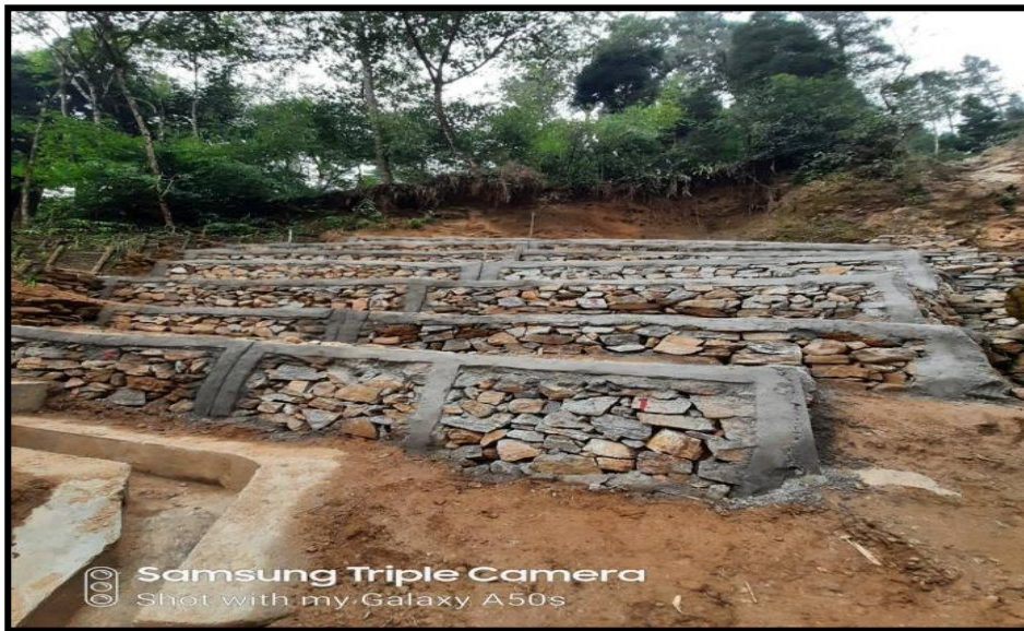
Hand packed wall of 150m 3 at Phuguri block constructed under RKVY during 2019-20 under West Balason Catchment Range of Kurseong Soil Conservation Division
