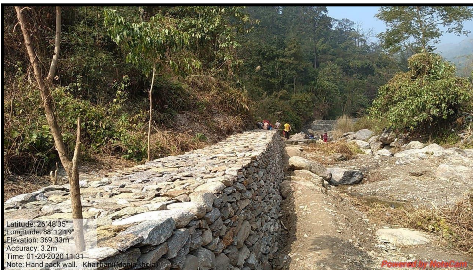
Hand packed wall of 100m 3 at Khairbani block constructed under RKVY during 2019-20 under Lower Mahandi Catchment Range of Kurseong Soil Conservation Division
