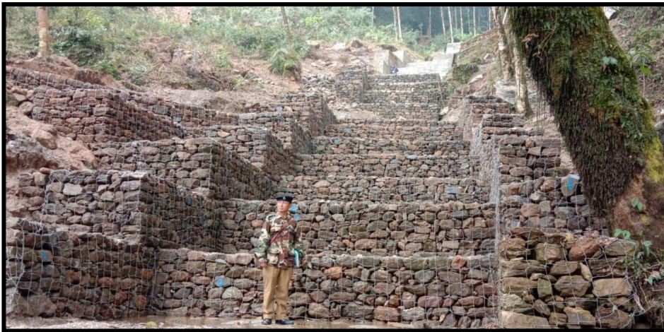
Boulder Sausage wall of 150m 3 at Mahaldiram block-II constructed under CAMPA FUND (TLDP-IV) during 2019-20 under East Balason Catchment Range of Kurseong Soil Conservation Division
